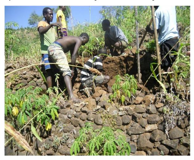
Figure 4-2: Stone terrace construction in the study area (Tamiru Karse2014)
