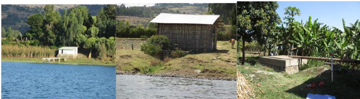
Figure 13: Lake water pumping projects at different wetland sites of Lake Lugo
