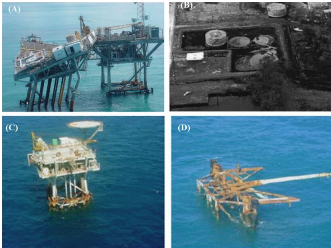
Figure 1. An extreme storm impacts on coastal and offshore petroleum infrastructure; (A) offshore platforms were damaged during a hurricane off of Louisiana [34]; (B) oil tanks were carried away by storm surge that caused over 1,750,000 L of oil release [35]; (C, D) before and after operating platform were destroyed during the 2005 hurricane season [36]
