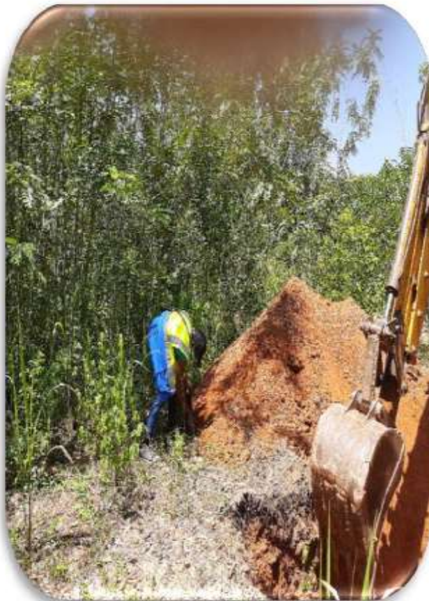
Figure 3.4: Material sampling in the excavated
