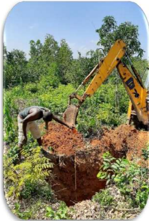
Figure 3.3: Trial pit being sunk
